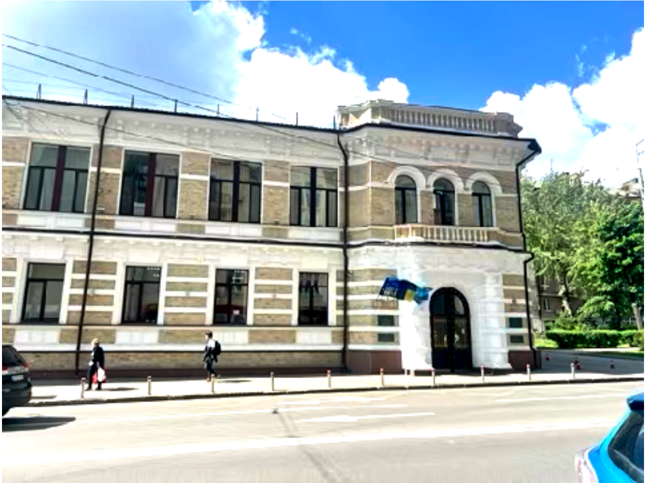
Figure 3 – former gymnasium building at Bulvarno-Kudriavska Street 18/2
