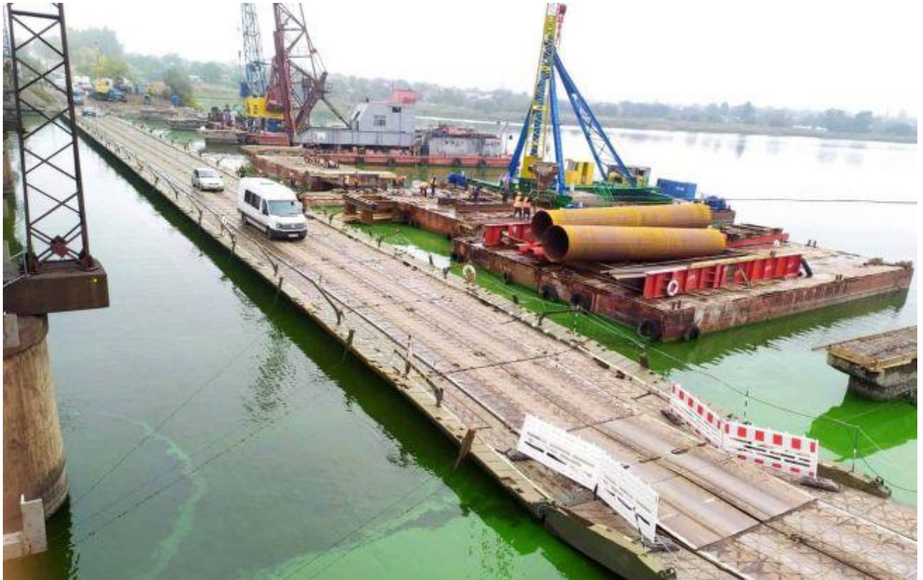
Figure 9 - Temporary pontoon bridge (Source: mil.in.ua)
