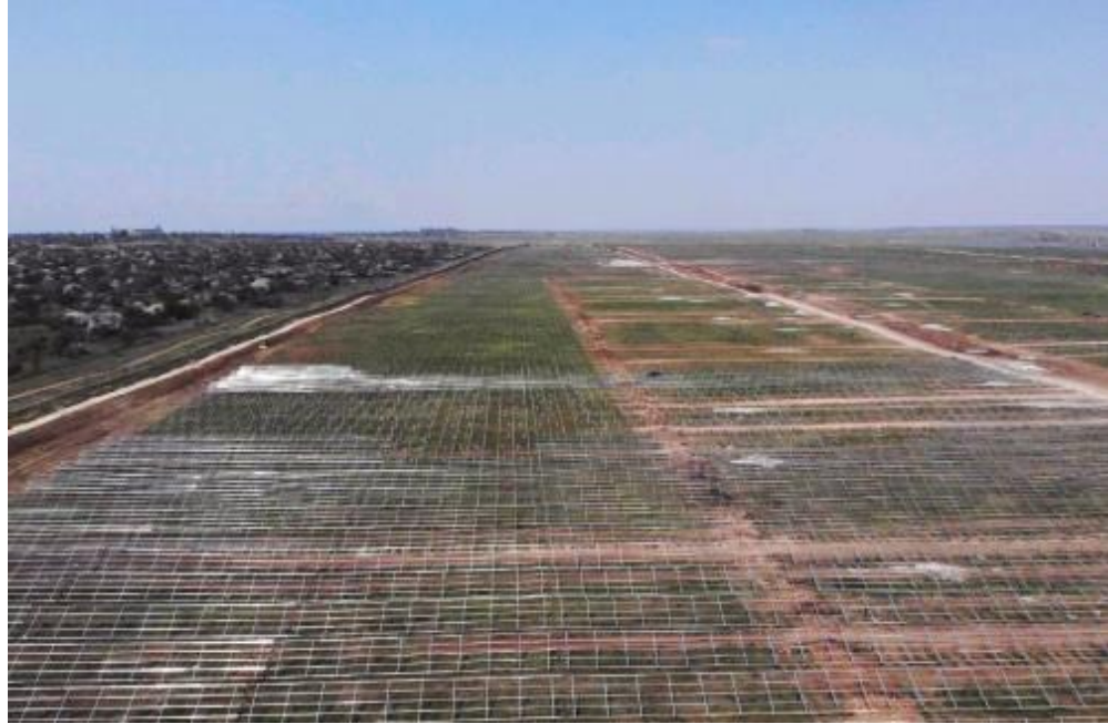
Picture 3. Pokrovska solar power plant in Dnipropetrovsk region
